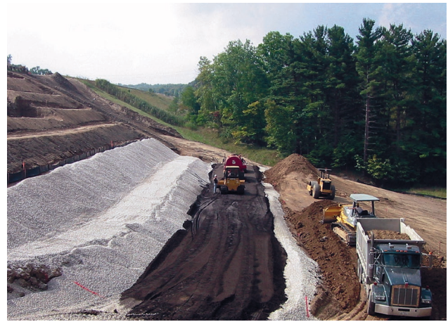
Figure 2. Example: Beneficial reuse of foundry sand on the Ohio Turnpike Project: (Photo courtesy of Kurtz Bros., Inc.)
