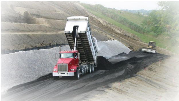
Figure 1. Example: Beneficial reuse of foundry sand on the Ohio Turnpike Project. (Photo courtesy of Kurtz Bros., Inc.)
